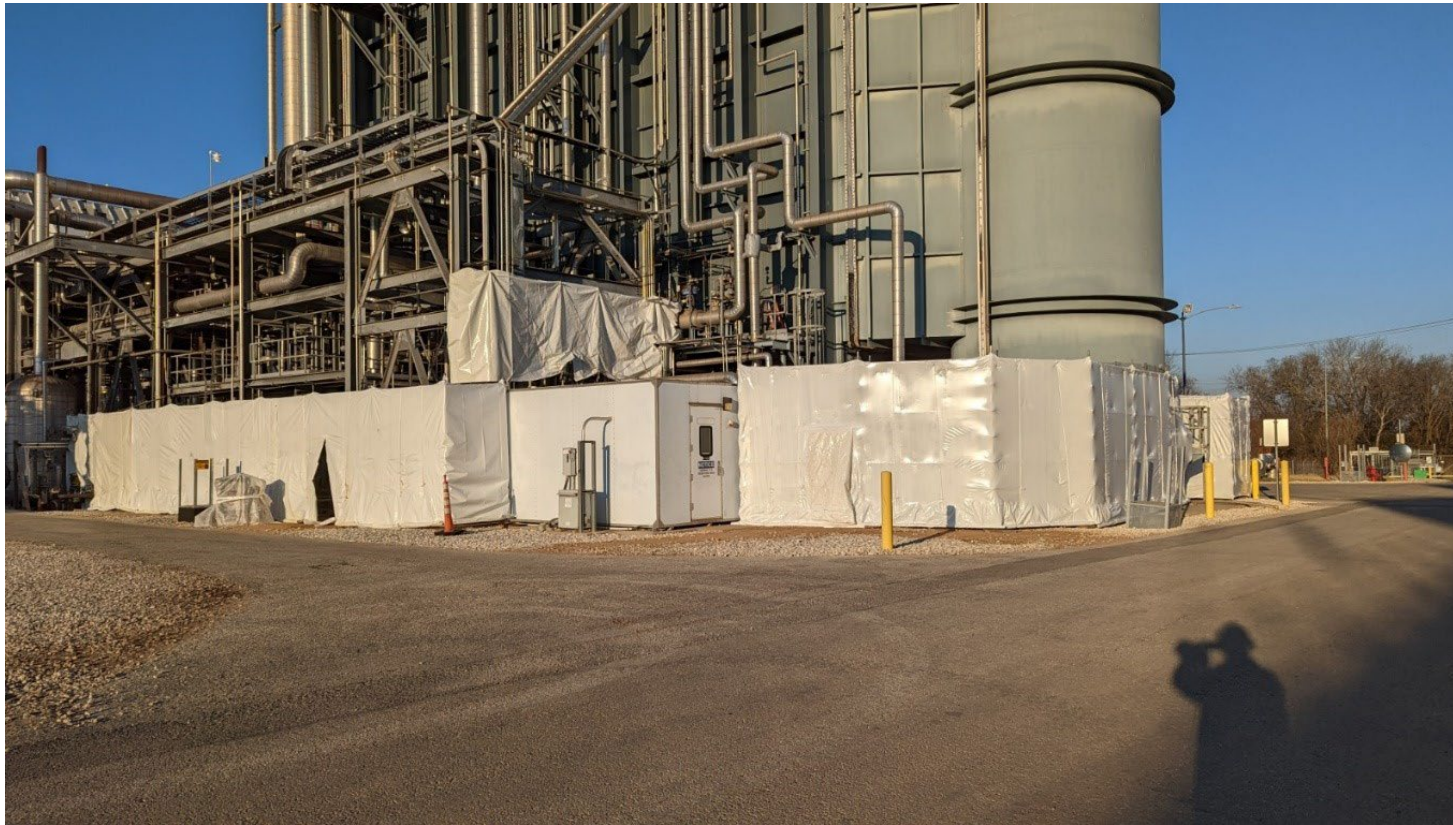
Left: HRSG ground level with completed wind walls.
