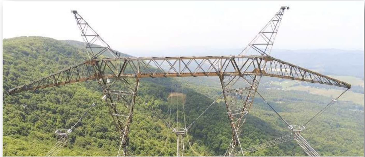
Polymer Suspension V-String Configuration
