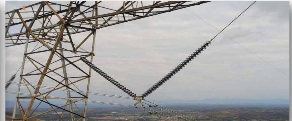
Ceramic Suspension V-String Configuration
