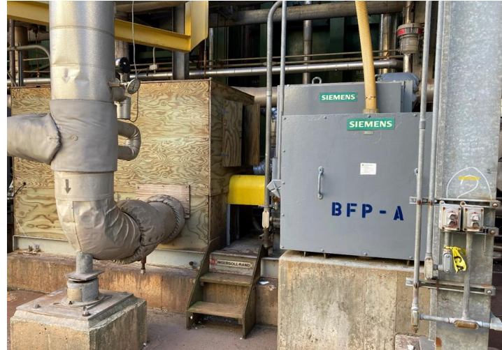
Fabricated Wood Enclosure (May include heat strips or lamps)
