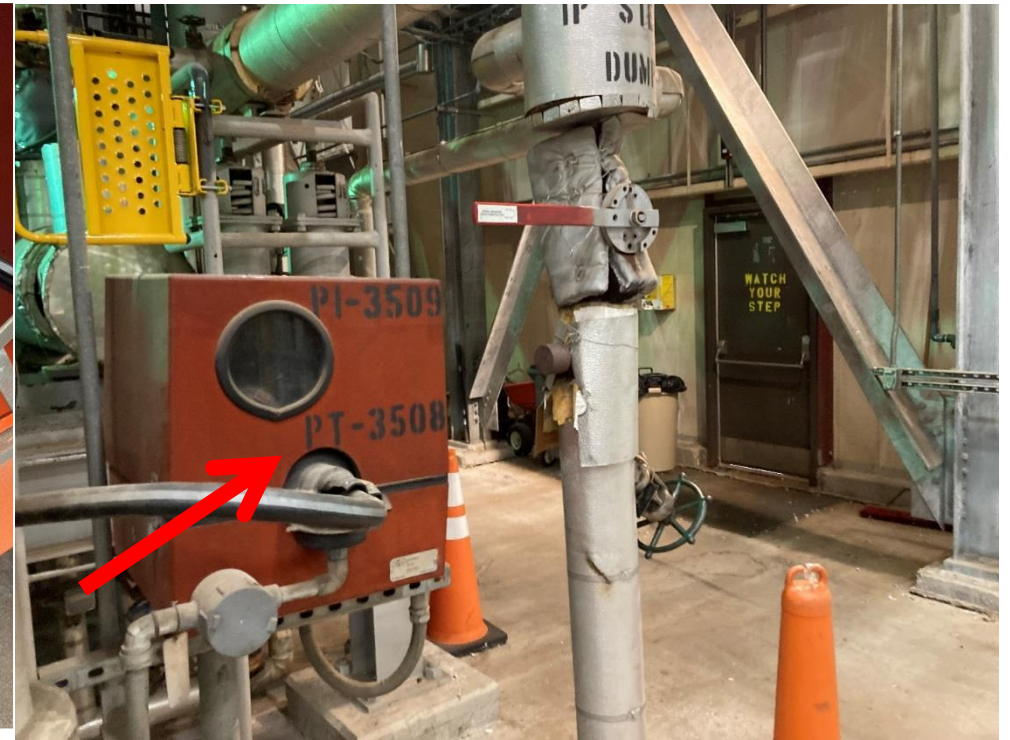
Heated Pressure Transmitter Enclosure
