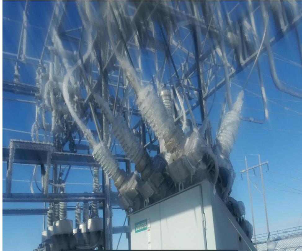
Frozen insulators can short equipment
